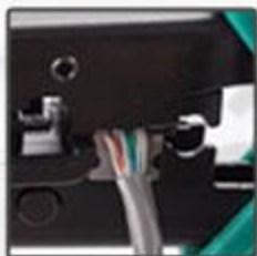
Stripping flat telephone cable
